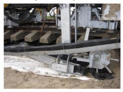
Figure 4 An example of an automated installation for laying geocells
